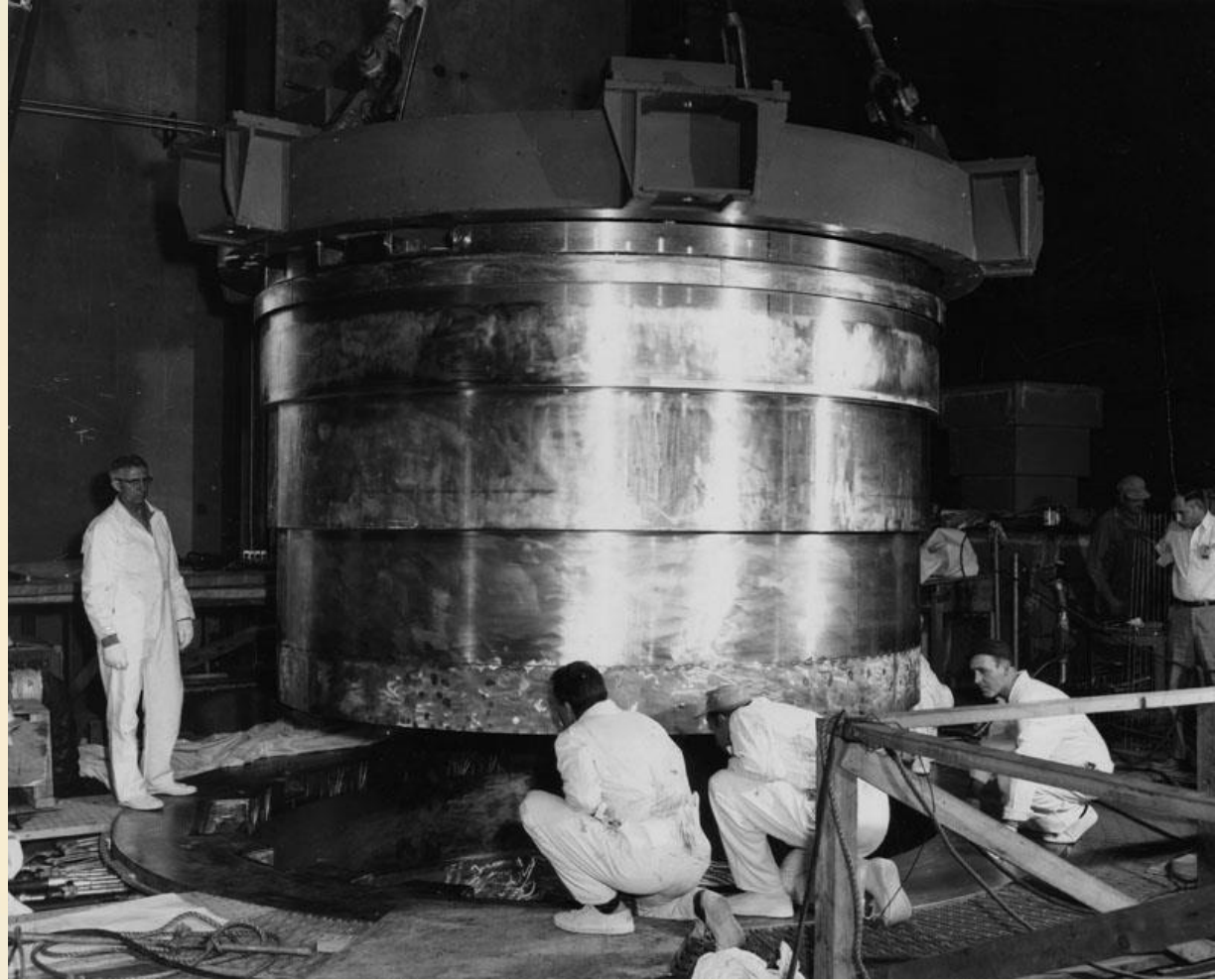
Installation of 75-ton shield, shield being lowered, for Sodium Reactor Experiment LAPL Valley Times Collection, 1957
