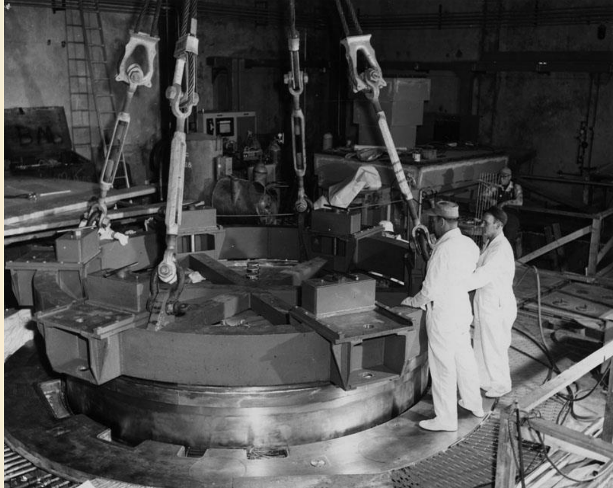
Installation of 75-ton shield for Sodium Reactor Experiment LAPL Valley Times Collection, 1957
